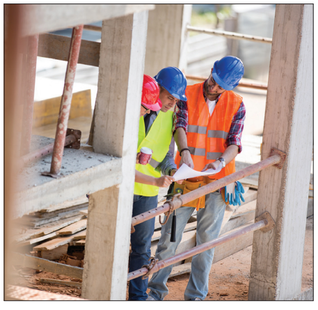
PHOTO COURTESY RSCCD COMMUNICATIONS The Rancho Santiago Community College District is committed to incorporating green design in new construction.
